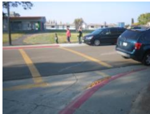
Additional red curb will help improve driver sightlines crosswalks adjacent to DH White
