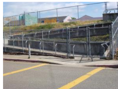
The rear gate at Matthew Turner is currently locked
