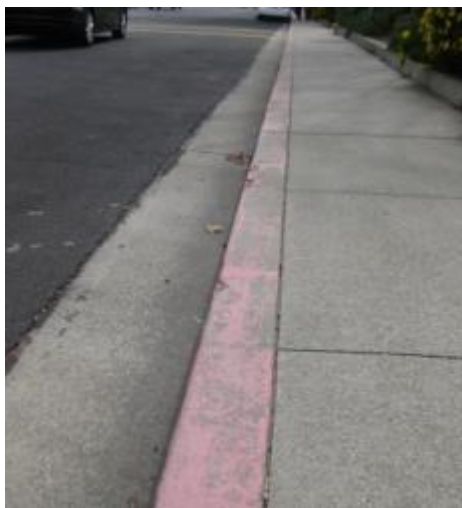
The red curb on Vanden Road needs refreshing
