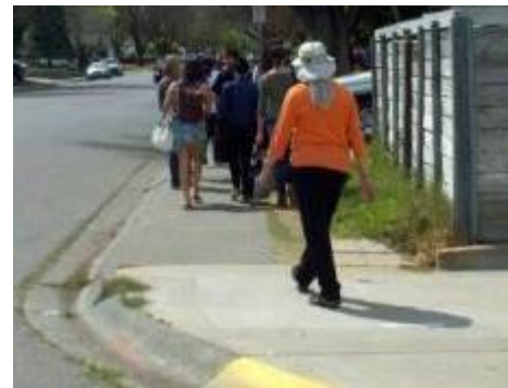
Students walking along a narrow sidewalk adjacent to a rolled curb
