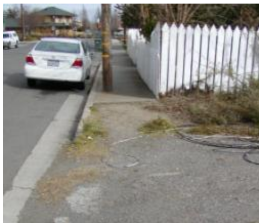
A sidewalk gap on the south side of West B Street, just east of North Adams Street
