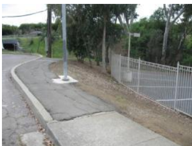
Sidewalk in need of repair leading to the pedestrian tunnel
