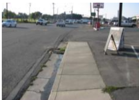
Sidewalks on State Route 12 are in poor condition
