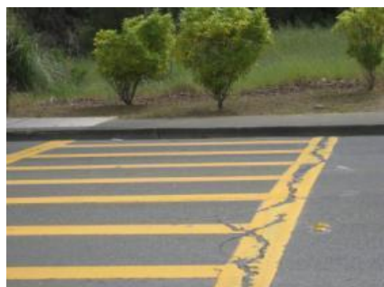
Missing curb ramp at Rose Drive
