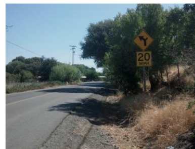
Montezuma Road sees high speeds coming into Rio Vista and lacks sidewalks from adjacent residential developments
