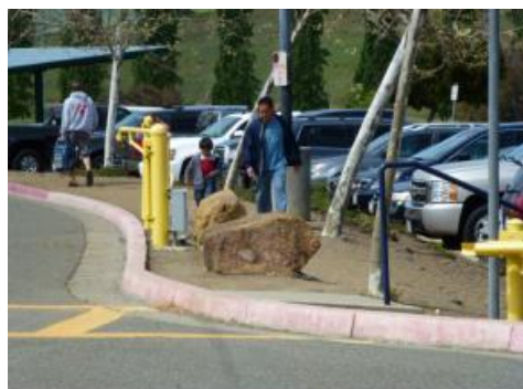
The crosswalk landing at Dempsey Drive needs improvements
