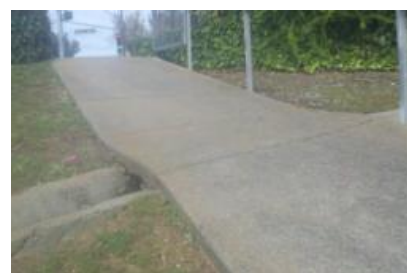
The current pedestrian path to 2 nd Street is not ADA compliant
