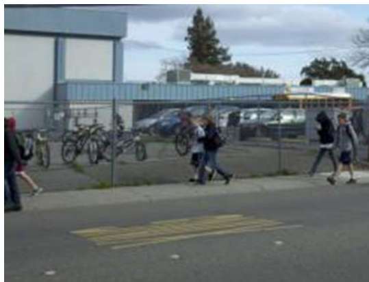
Narrow sidewalks on North Lincoln Street force students to walk in the roadway
