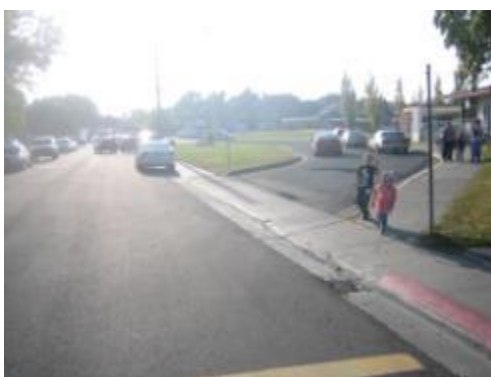
The Laurel Way crosswalk doesn't meet properly with the sidewalk on the loading loop
