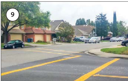
Curb ramps not aligned to crosswalk a the Vanden Road and Marshall Road intersection.
