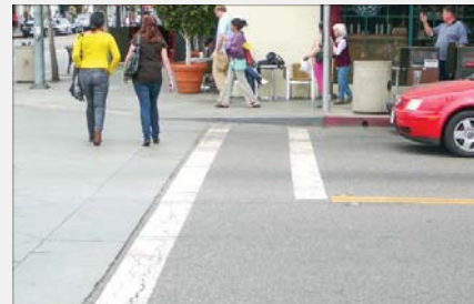
Stop bars set back from crosswalk provide additional buffer between vehicular traffic and pedestrians.
