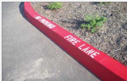
Red curb paint designates areas where parking is prohibited.
