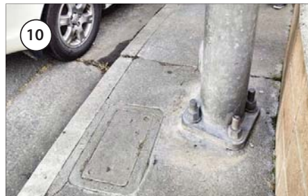
10 At the intersection of E Tabor and Dover, there are 3 obstructions. These exist on the NW, NE, and SW legs. Obstructions in the sidewalks include poles reducing the width of the sidewalk, like the one picture above on the NE corner.
