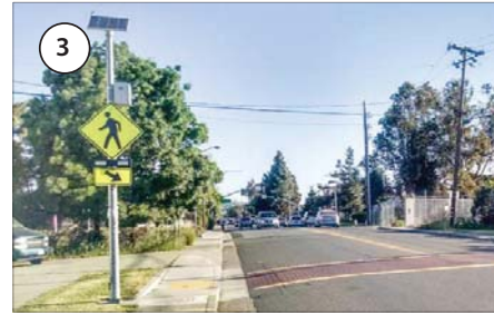
3 Rectangular Rapid Flashing Beacon at the intersection of Dover Avenue and Nightingale Drive.
