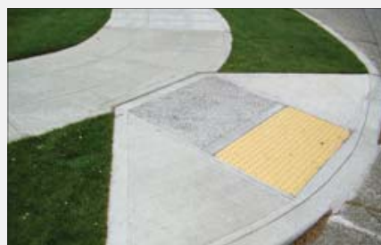
Curb ramps provide access to disabled pedestrians and parents walking with strollers.
