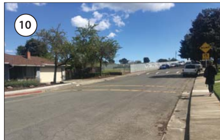
Existing crosswalk along Las Palmas Avenue is transverse and difficult to see, and lacks school area crossing signage and ADA-compliant curb ramps.
