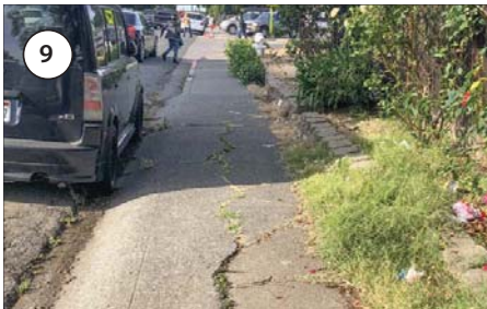
Cracked sidewalks near school present potential tripping and accessibility hazards.
