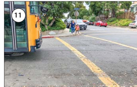
Existing crosswalk at the Carolina Street and Sutter Street intersection lacks high visibility markings and advanced stop bars.
