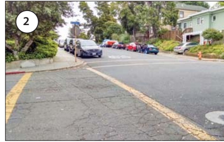
Corner curbs at the intersection of Carolina and Sutter Street lack curb ramps and sufficient red striping.
