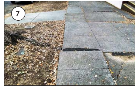
Existing sidewalks along Carolina Street feature cracked and uneven paving and present potential tripping hazards.
