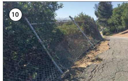
Multi-use pathway that parallels to Military West features cracked sidewalk, overgrown landscaping, and deteriorating fence.
