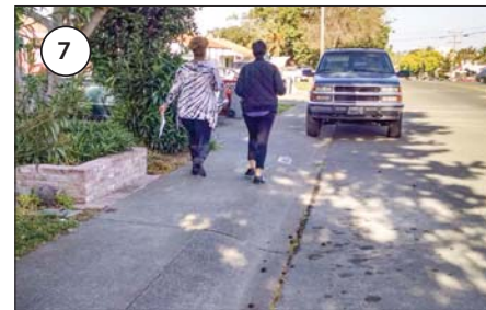
Sidewalk along Georgia Street features rolled curbs.
