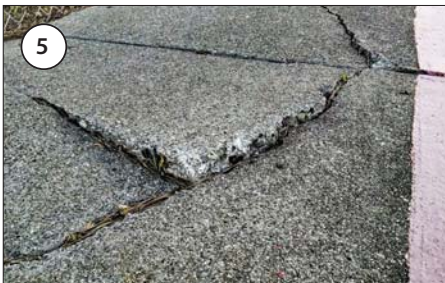
Cracked and uneven paving along nearby sidewalks present potential tripping hazards for pedestrians.
