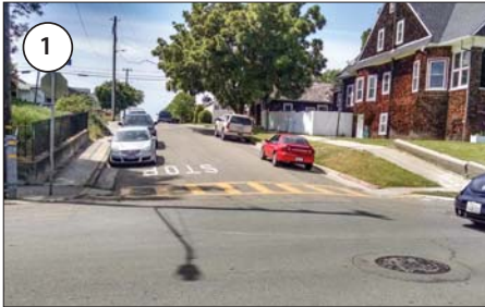
Crosswalk at intersection of 2nd and Santa Clara lacks adequate surrounding red curb striping.
