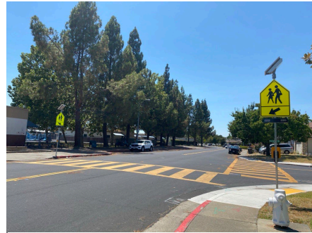
Completed RRFB installation at Cement Hill Road
